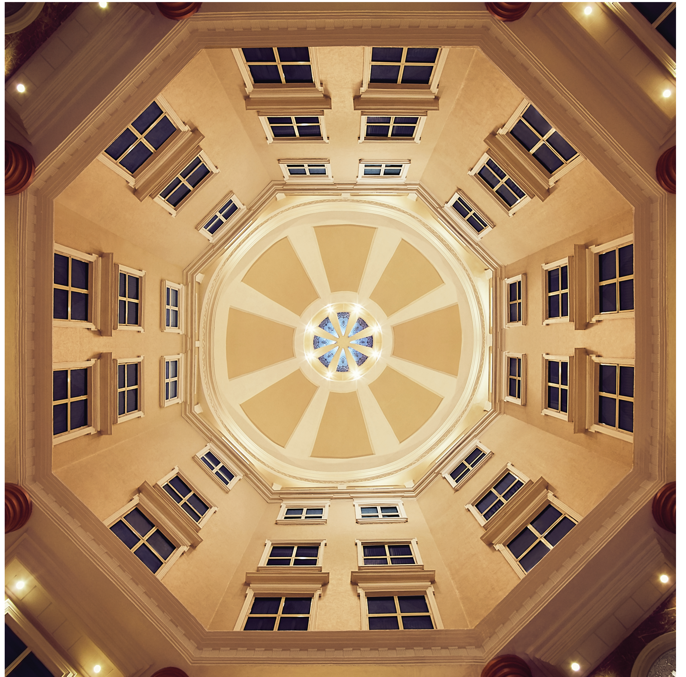
Interior image of Olympia, Hiranandani Gardens, Powai.
